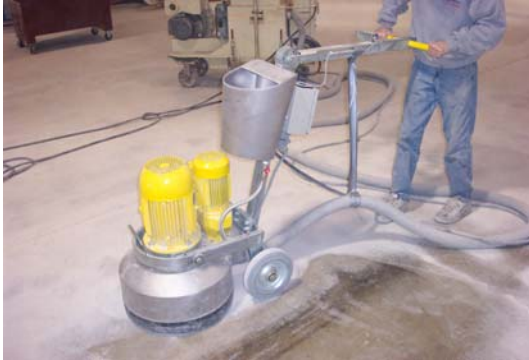
Concrete Grinding
