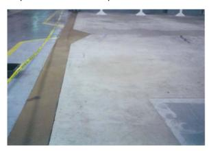
Another common problem is irregular transitions in slabs. They can cause damage to equipment product and pose a danger for lift operators. Transitions are repaired by using a high strength repair mortar to feather off high edges and provide a smooth rolling surface. Your employees will really appreciate these types of repairs.
