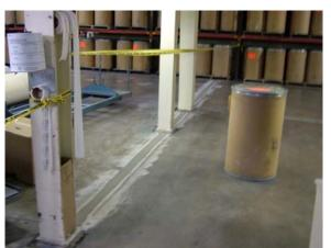
Many times, large expansion joints in floors become a rolling load problem; they can tip or cause product to shift. These large joints can be properly prepared and filled with a semi flexible repair mortar to product a smooth transition from one side to the other. These types of repairs will make traveling over these "hard to get over" spots a thing of the past and will improve
