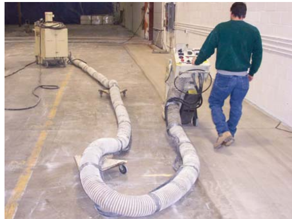
Removing acrylic sealer
