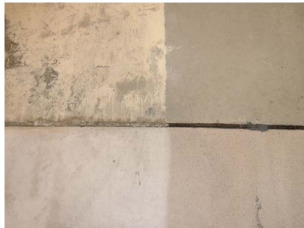
Removing paint
