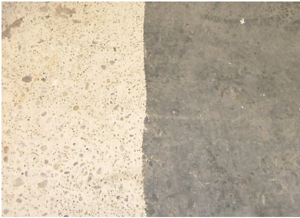
Removing dirt and oil
