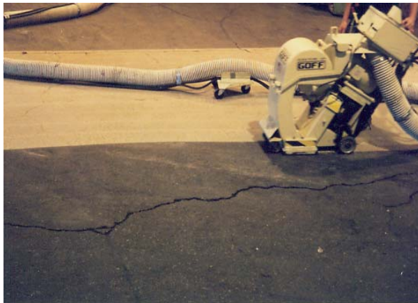
Preparing dirty concrete
