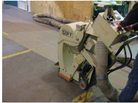
Preparing for coating
