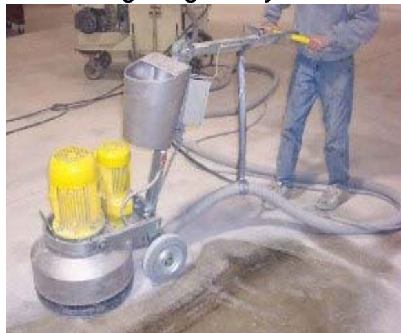
Concrete Grinding
